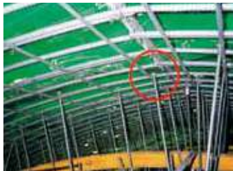
Reinforcement for tunnel covering
