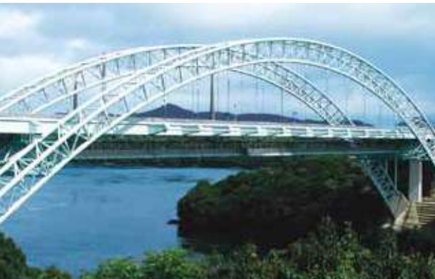
Sea bridge using high-frequency bending technology
