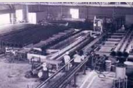
Straight pipe lining (1971)
