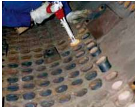
Boiler tube removal (Induction heating tube shrinker)
