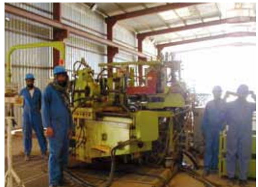
On-site bending (Middle East)
