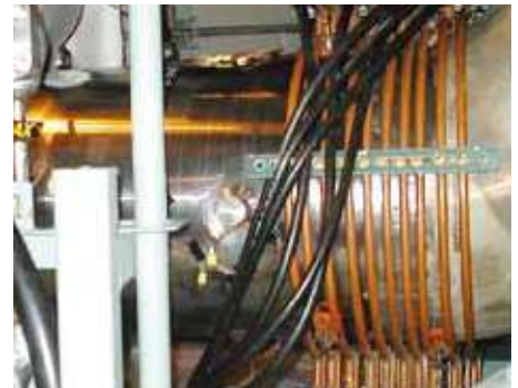
Induction Heating Stress Improvement (IHSI)
