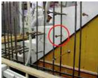
Fixture of precast stair reinforcement
