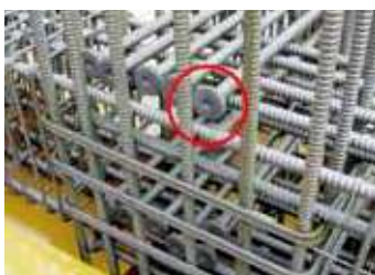
Fixture of beam reinforcement
