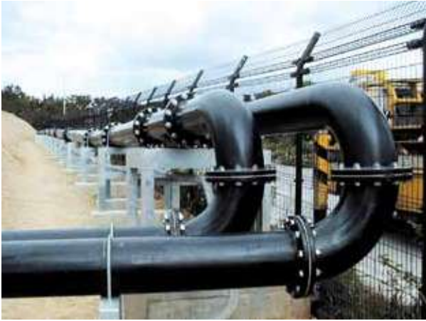
Polyethylene pipe lining (inside and out)
