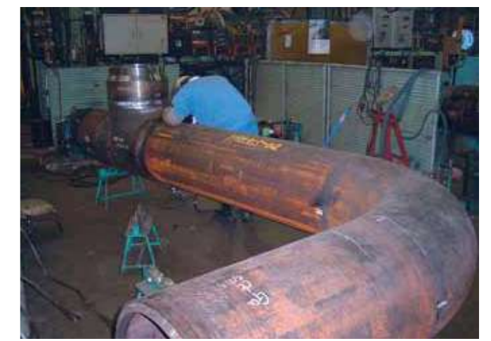
Welding service for Power plant piping
