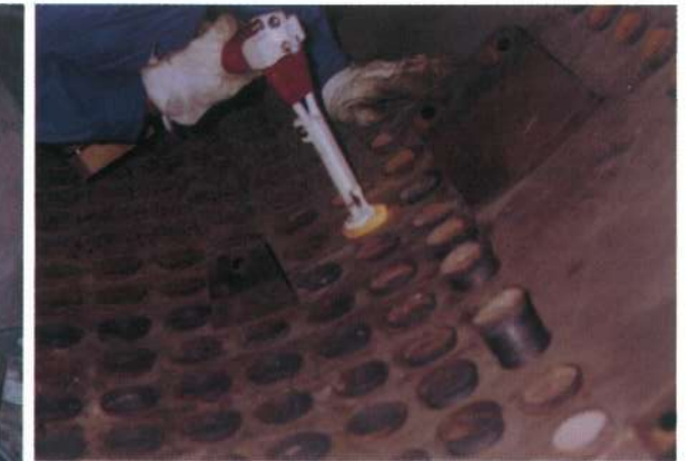
抜管 Tube Removal
